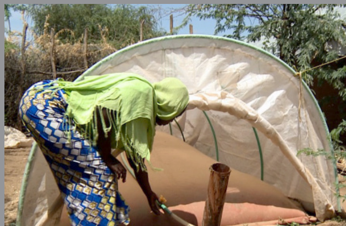
Naimana inspects her biogas digester, which uses waste from livestock to generate biogas.
