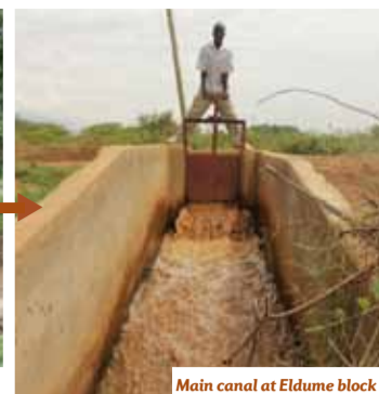
Main canal at Eldume block
