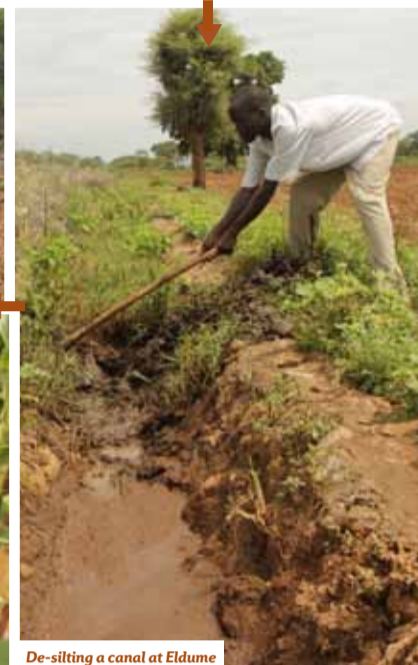
De-silting a canal at Eldume
