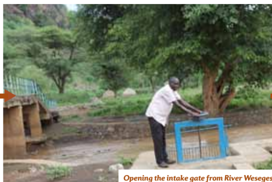
Opening the intake gate from River Weseges
